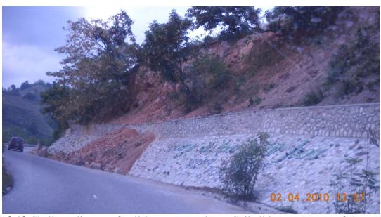
**Figure 9.12** Shallow slip-out of soil in upper road cut. Soil slid over the top of the surviving masonry wall and slope protection. (N18.440270, W72.636207).
