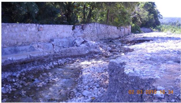
**Figure 7.12**. Damage to stone wall resulting from lateral spreading. Note the surficial cobbly material revealed by the failure scarp in the foreground. (18°25'33.31"N, 72°43'34.58"W looking southward away from coast).
