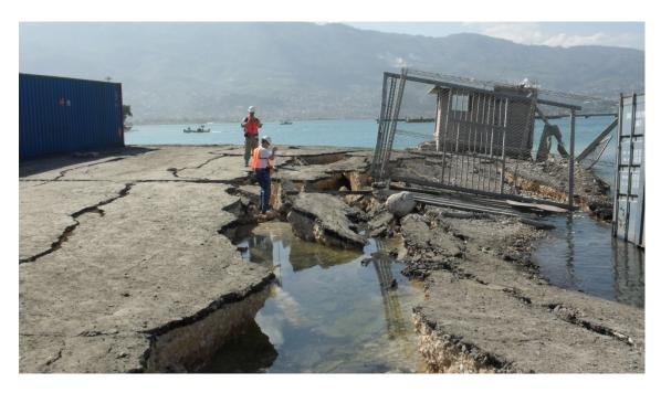
**Figure 6.9** Lateral spreading west of the two metal warehouses. Photo taken facing south with the metal warehouses to the left. (N18.557075, W72.352045)
