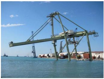
**Figure 6.12** Submerged 15-m gauge container crane (foreground) and mobile crane (background). Photo taken facing west. (N18.55598, W72.348564)
