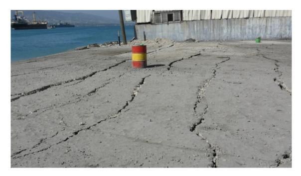
**Figure 6.7** Lateral spreading between the two metal warehouses, adjacent to the collapsed North wharf (left). A cumulative total of 89 cm of horizontal movement (determined by crack width) was measured in a zone extending inland approximately 30 m from the post-earthquake shoreline. Post-earthquake imagery indicates lateral spread cracking extended 50 m inland. (N18.556696, W72.34787)
