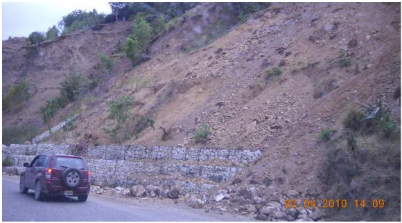
**Figure 9.10** Shallow rock topple or rock fall from over-steepened road cut. Debris slid over the top of stable gabions at the toe of the slope. (N18.409159, W72.638815).
