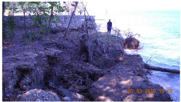
**Figure 7.11**. Damage to stone wall resulting from coastal failure and lateral spreading. (18°25'33.94"N, 72°43'34.27"W looking westward).
