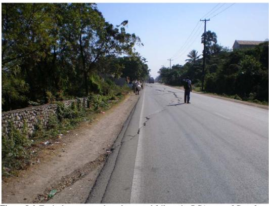
Figure 8.4 Typical arcuate road cracks at road failure site RCA west of Carrefour.
