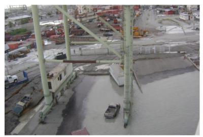
**Figure 6.13** Photo taken immediately after the earthquake with the crane in its most eastward position and with the landside legs of the crane above water. Photo taken facing east. Source: unknown (N 18.556056, W72.347981)
