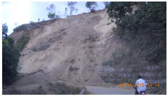
**Figure 9.11** Relatively shallow slip-out of regolith. Disaggregated material flowed over stable gabions ands blocked over half the road. (N 18.409159, W72.638815).
