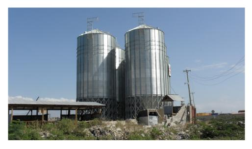
**Figure 6.19** Post-earthquake photo of steel grain hopper silos (photo taken facing North). The silos showed no visible signs of distress. (N18.558431, W72.350350)
