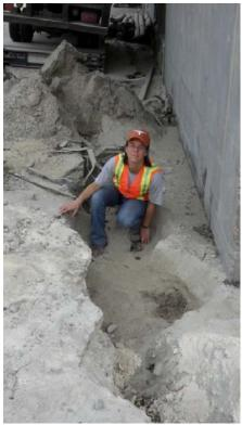
**Figure 6.10** Liquefaction and lateral spreading adjacent to the north side of the metal warehouses. Photo on top taken facing west, photo on bottom taken facing east. (N18.556961, W72.349751)
