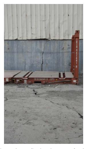
**Figure 6.11** Lateral spreading crack extending into the western foundation wall of the west warehouse. Photo taken facing east. (N18.55721, W72.35179)
