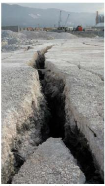
**Figure 6.22** Lateral spreading in the storage yards in the northern part of the port facility. Photo taken facing South. (18°33'41.76"N 72°20'52.25"W)
