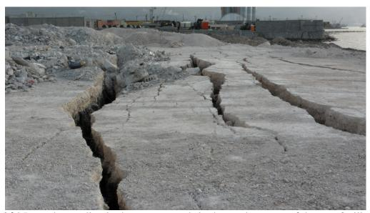
**Figure 6.21** Lateral spreading in the storage yards in the northern part of the port facility. Photo taken facing South. (18°33'41.39"N 72°20'52.51"W)
