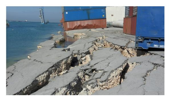
**Figure 6.6** Lateral spreading adjacent to the collapsed North wharf. Note the crane in the water in the background and the metal warehouses on the right. (N18.55622, W72.34787)
