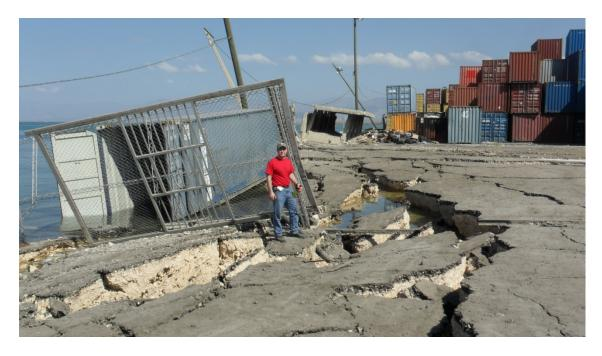
**Figure 6.8** Lateral spreading west of the two metal warehouses. Photo taken facing north with the metal warehouses to the right. (N18.557075, W72.352045)
