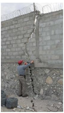
**Figure 6.23** Lateral spreading in the storage yards in the northern part of the port facility. Lateral spread crack passes through a stone/masonry wall. Photo taken facing South. (Approximate long. and lat. of photo: 18°33'35.15"N 72°20'56.18"W)
