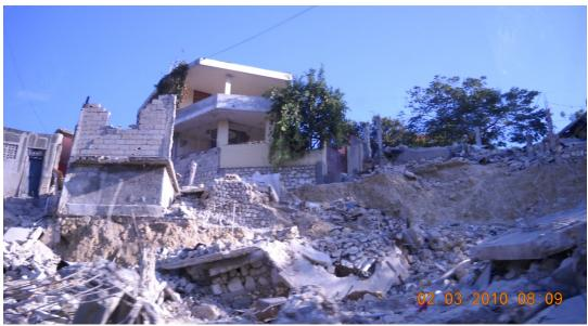
**Figure 9.7** Several buildings have collapsed in this location. Although there are scarp-like near vertical surfaces near the top of slope that may suggest the possibility of a deeper rotation failure, in our opinion the observed conditions are likely due movement of soils adjacent to failed walls, as discussed in the text. (N18.528406, W72.309920).
