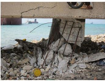
**Figure 6.16**: (top) Damage to piles supporting the pedestrian bridge connecting the South Pier to the island (photo taken facing South) and (bottom) extensive damage to the landward row of piles (photo taken facing West) (N18.554628, W72.351492)
