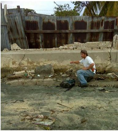
**Figure 4.16**. Water mark for high tides on sea wall at Ca Ira, Léogâne. Residents indicate high tides no longer extend up the wall to the former high tide level (N18.524924, W72.650871)
