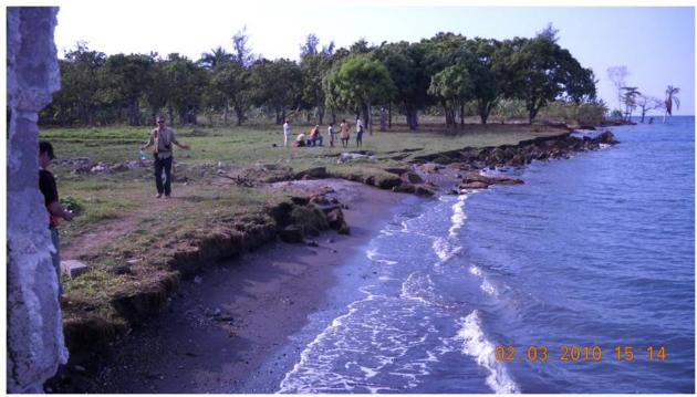
**Figure 7.17**. Scarp formed along northern portion of coastal failure near village of Grand Goâve. (18°25'53.82"N, 72°45'37.16"W looking northwest).
