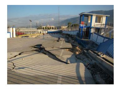
**Figure 6.25**: Damage to entrance road caused by lateral spreading. Photo taken facing South-East. (Approximate long. and lat. of photo: 18°33'11.61"N 72°20'52.50"W)
