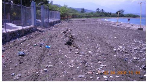
**Figure 7.5**. Ground cracking along coastline near village of L'Acul. (18°26'48.83"N, 72°41'11.39"W looking west).
