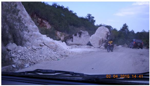
**Figure 9.8** Topple or fall included several large boulders in this old quarry. (N18.439010, W72.646168).
