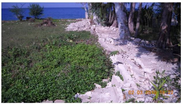
**Figure 7.20**. Damage to unreinforced block wall running perpendicular to coast near village of Grand Goâve. (18°25'51.84"N, 72°45'38.06"W looking northeast).
